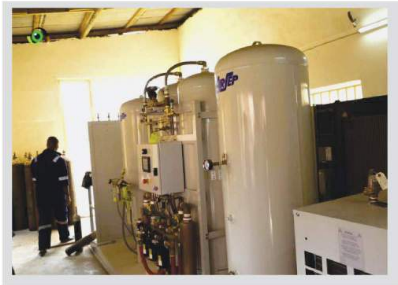
The oxygen generation plant installed by the new administration generates enough oxygen for the hospital use. Photo credit: Nigeria Health Watch
