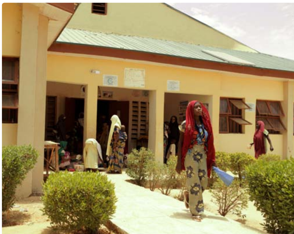
Refurbished health facility
