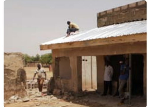
Repairing a health facility in the north
