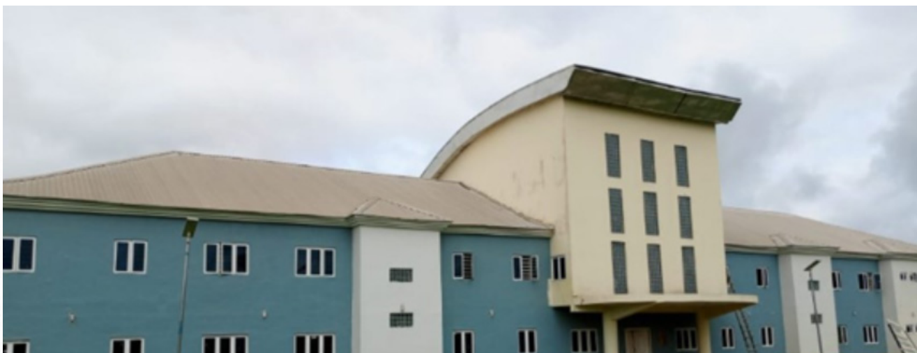
Completion of the New General Outpatient Department Complex, Irrua Specialist Teaching Hospital, Edo State.
