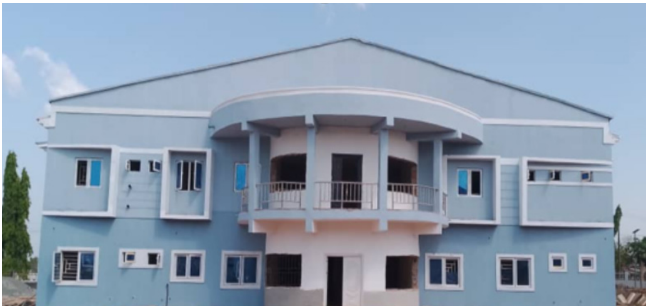
Near completion of the Children's Emergency Ward, Irrua Specialist Teaching Hospital, Edo State.
