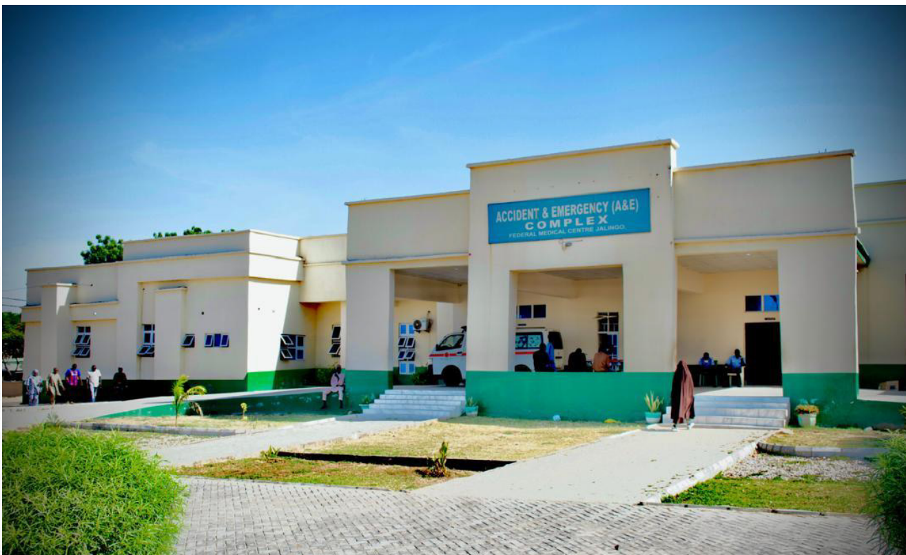
Recently completed accident & emergency, Federal Medical Center , Jalingo Taraba State.
