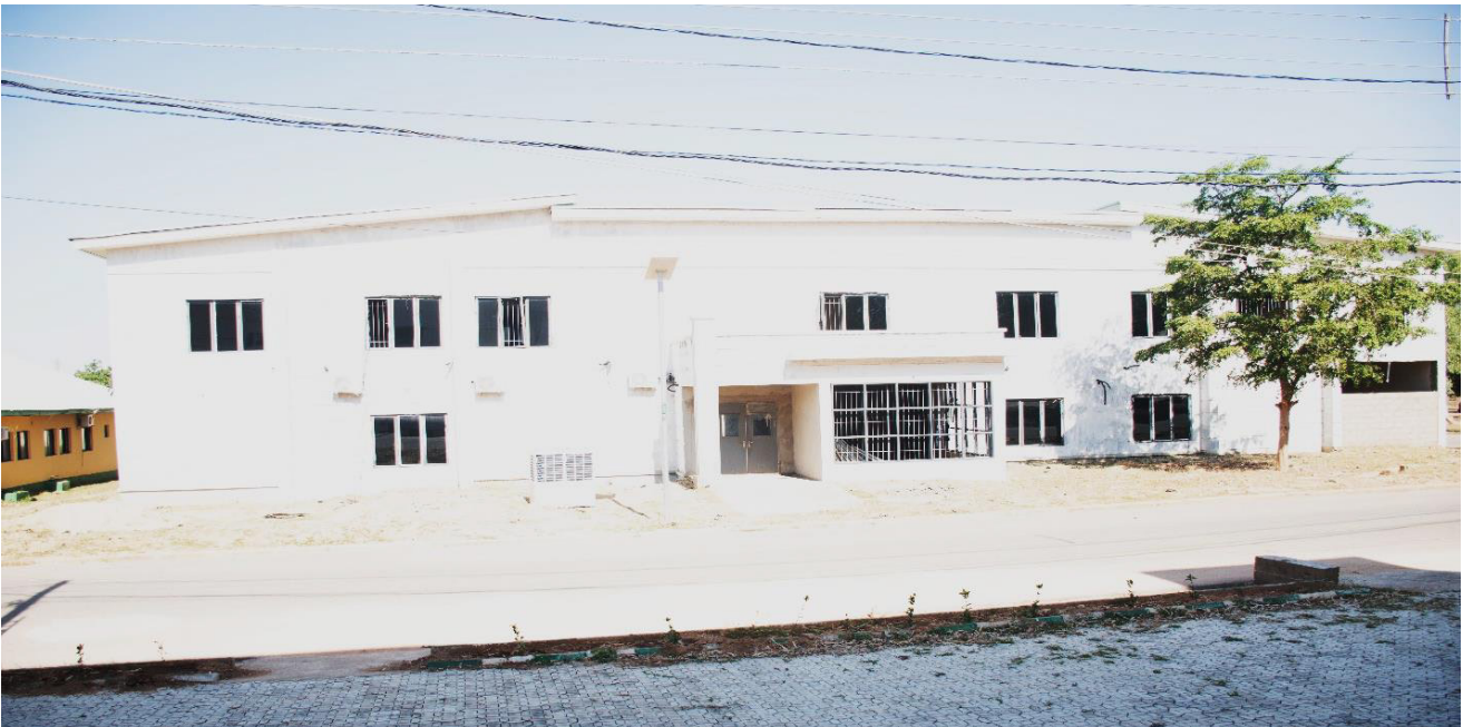
Ongoing imaging center, Federal Medical Center, Jalingo Taraba State.
