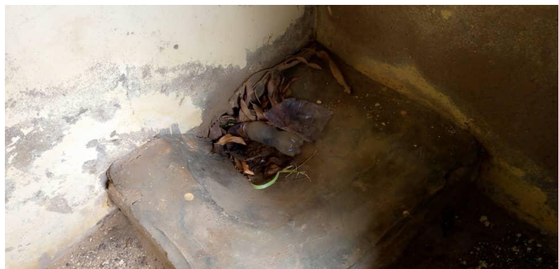
Inside the toilets of Government Girls Secondary School Lemu with a student population of over 1000
