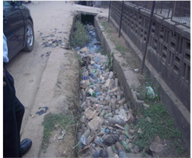
Figure 3: blocked drains as a result of abuse of drains with waste deposits
