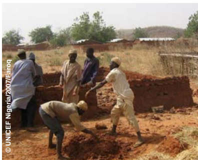
School based management committee members of Dagwarga Ubandawaki building a library for the school.
